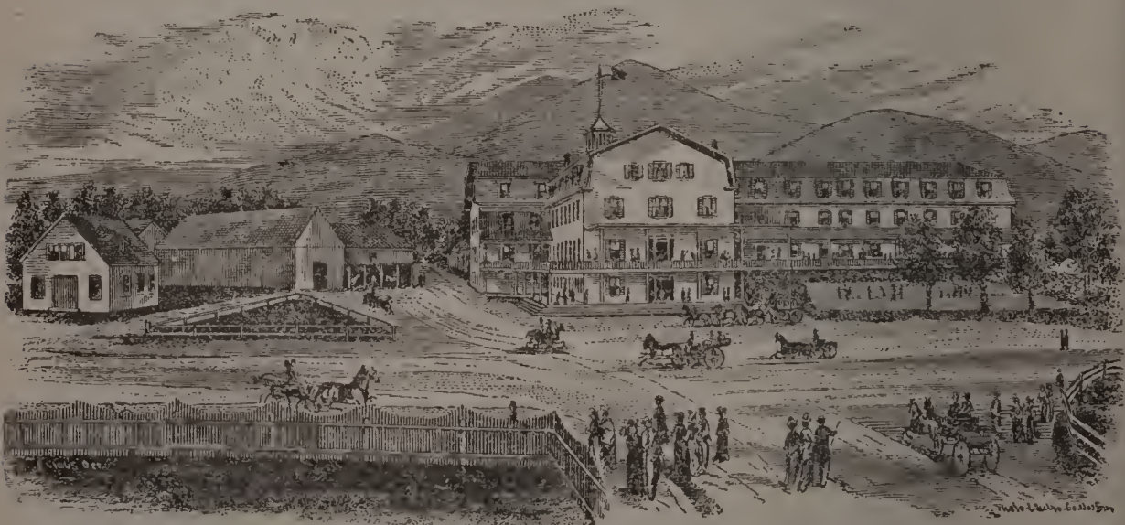
WAUMBEC HOUSE, JEFFERSON HILLS.
